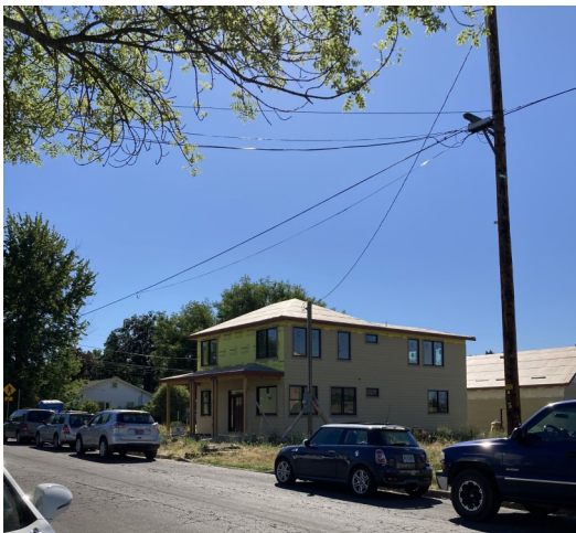
Jackson County Fuel Committee's new building across the street from the church, rising out of the ashes of it's previous housing.
